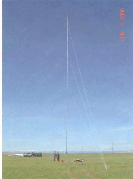
Figure 2 30-meter tower installed on the Rexburg Bench
